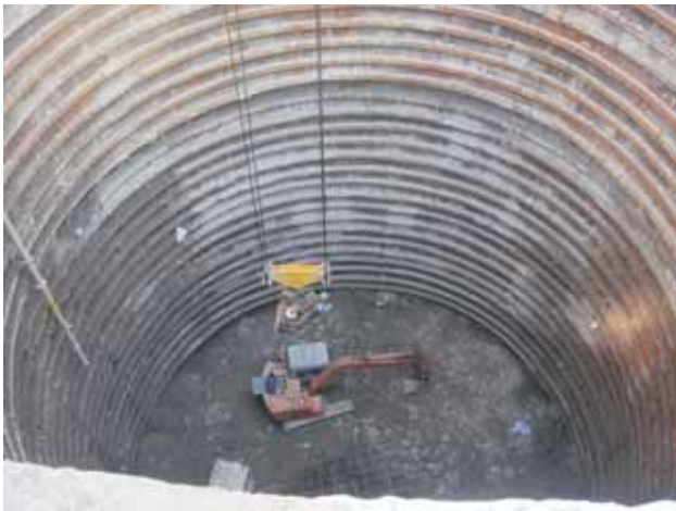
Vertical Surge Shaft of 14 Mtrs. Dia and Height of 77 Mtrs. With complete RIB support.
