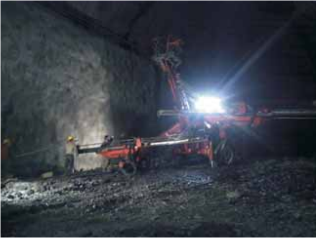
Double Boom Tamrock working in Power House Cavern fixing Rock Bolts.
