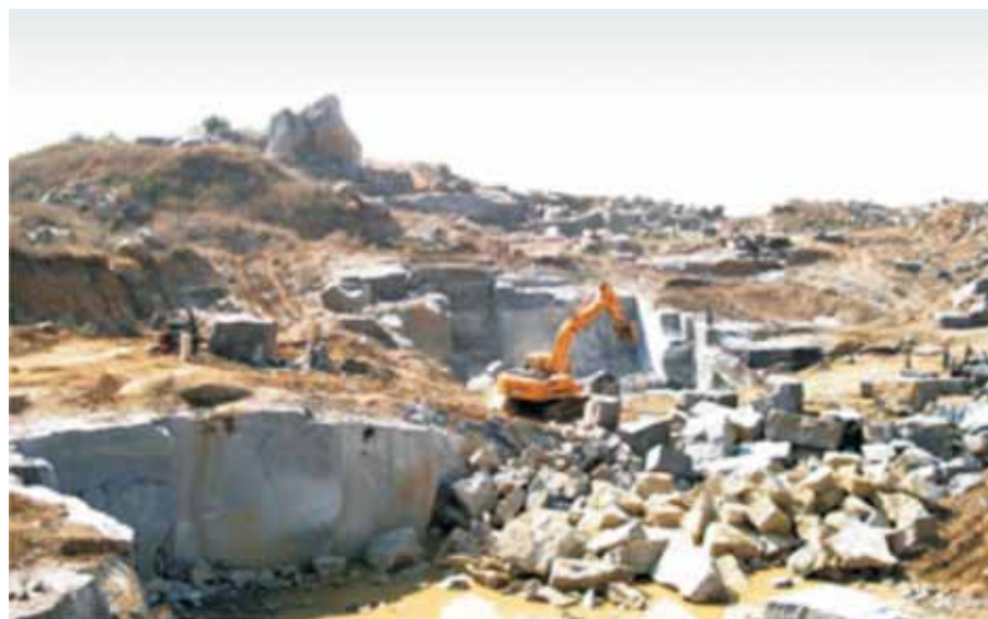
ROUGH GRANITE BLOCKS QUARRIED FROM OUR INDIAN AURORA QUARRY -BHEEMGAL, NIZAMABAD DISTRICT
